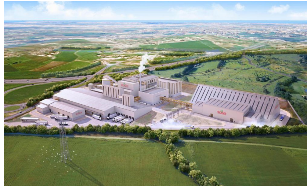
Sugar Refinery, Algeria
