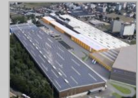
SEK 17 m Order Building Systems, Switzerland, and 3 more above SEK 10 m in the quarter (Africa, Poland and Germany)
