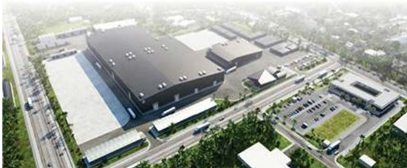
Multi purpose facility, Calabar, Nigeria
