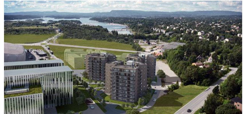
Fornebu Construction project in Norway
